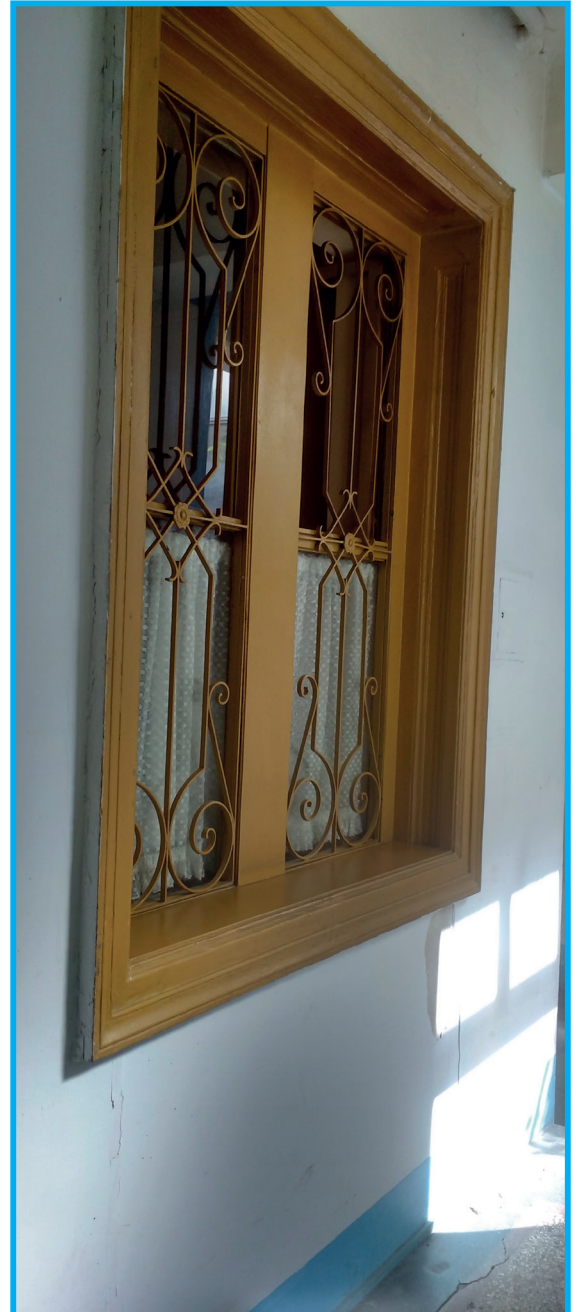
Fenster am Gang
